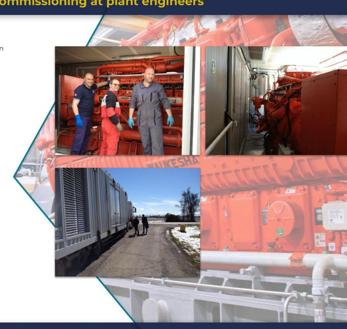
Rio Marsilia landfill, customer of MTM energia srl, with a TEDOM TB110G5VN7X86 engine for self-generation of energy consumption at the landfill, rated at 100 KWe.
