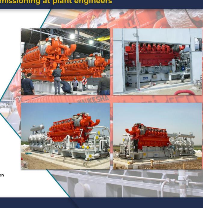
Our second project was the APG 1,000 for Bi which is a biogas-fed cogeneration plant using poultry manure. Again, it involved a 1 MWe Waukesha engine.
